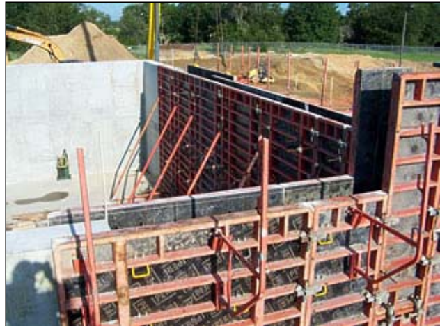
Construction at a water supply development project.
