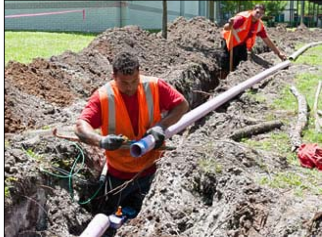
Purple piping is installed to extend a reclaimed water line.
