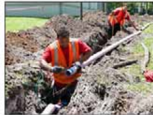
Pipes going to be installed to extend a reclaimed water line
